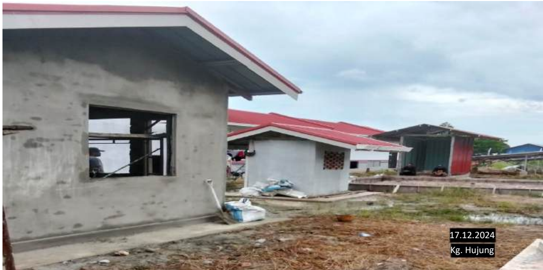
b) Ancillary Building & Skid Tank
