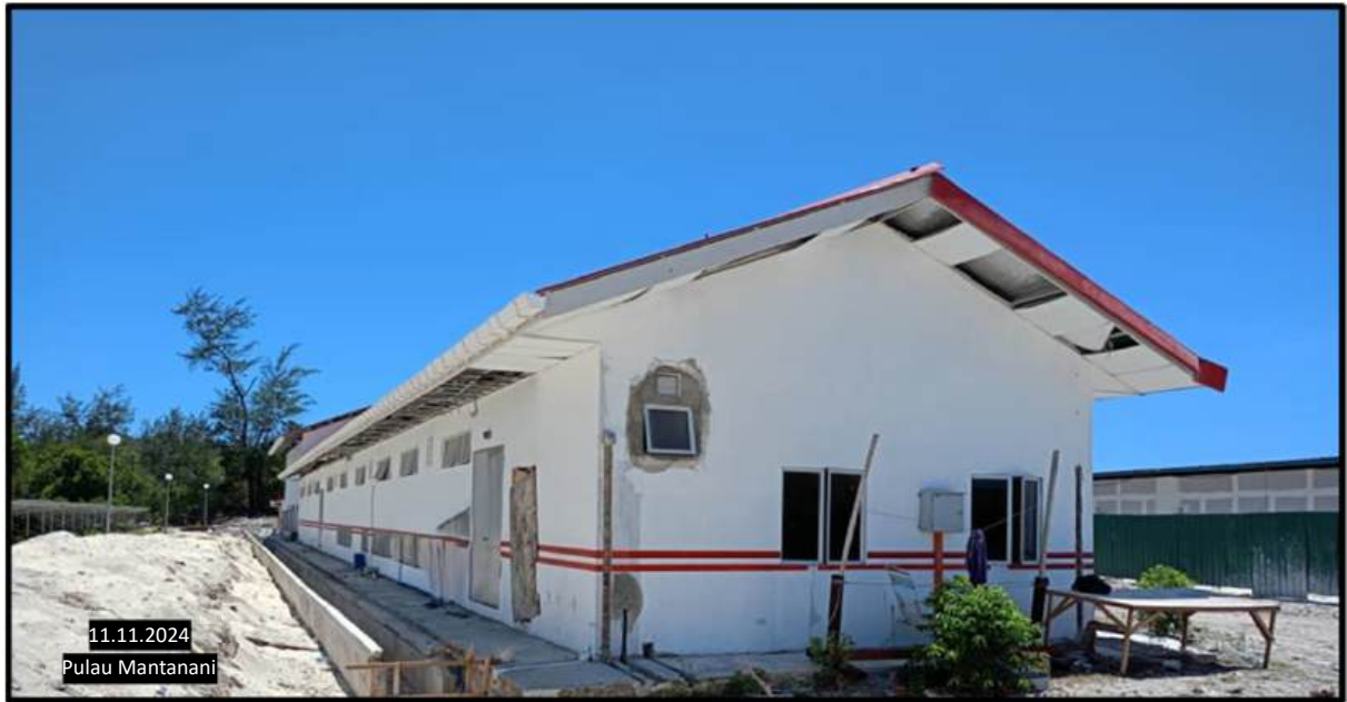
a) Power House Building
