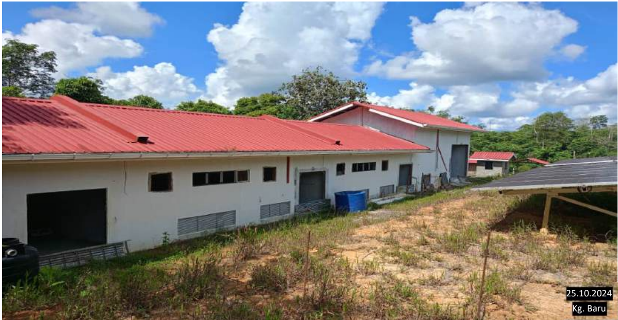
a) Power House Building
