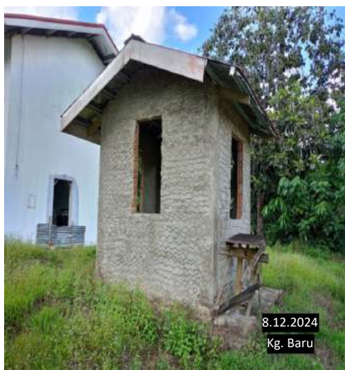
b) Ancillary Building
