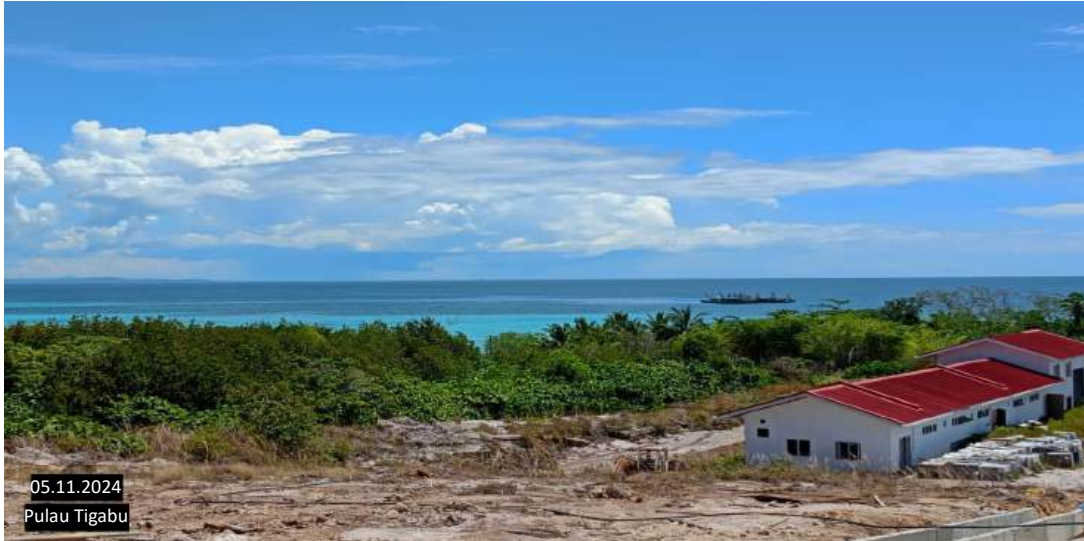
a) Power House Building
